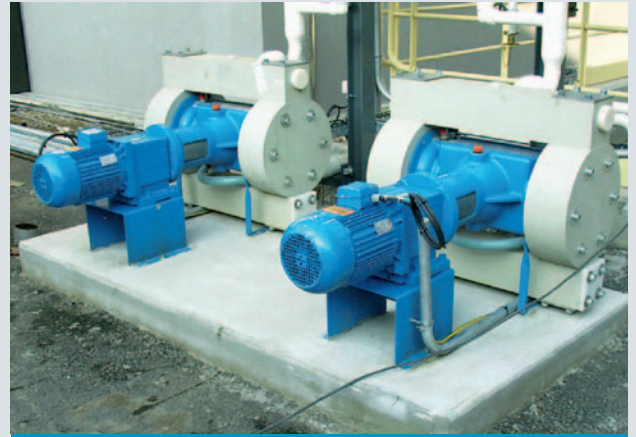
EM-050-PP for transfer of acidic waste water in the chemical industry
