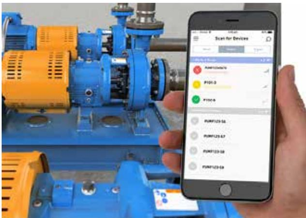
Spend less time collecting data and more time fixing problems. The i-ALERT<sup>®</sup>2 mobile app has the ability to scan multiple i-ALERT<sup>®</sup>2s within range to quickly and safely inspect multiple machines.
